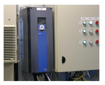
A VACON 100 HVAC drive at Meri-Lapin Vesi Oy's water intake plant. The VACON 100 HVAC drives are also available in IP54 enclosures, which can be installed directly on the wall at the plant. This brings space and cost savings. A high resolution graphic panel and installation wizard improve user-friendliness during installation and daily operation. Built-in fieldbus connections bring savings in investment costs.
