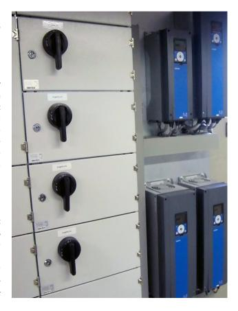
VACON 100 FLOW units at the Osvald waste water pumping station. The drives were installed on a backplate at SK-kojeisto, the Seinäjoki, Finland based company that has built the switchboards used at KRS-Vesi.
